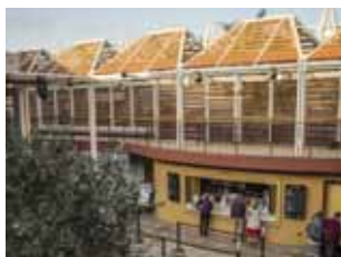
The Conrad Prebys Performing Arts Center, La Jolla, CA. Epstein Joslin Architects, Cambridge, MA Seite / Page 136
